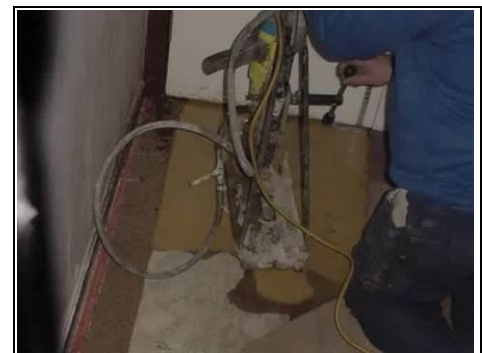
Example of first core sample being taken from the basement
