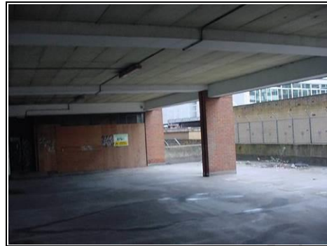
Concrete frame visible to basement area
