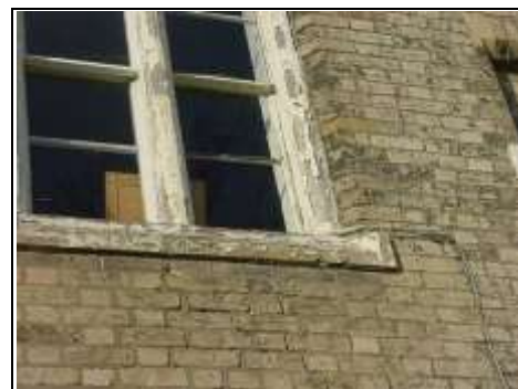
Paint flaking off rear windows, bare timber visible
