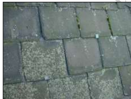
Close up of slates showing lead tingles to front of building
