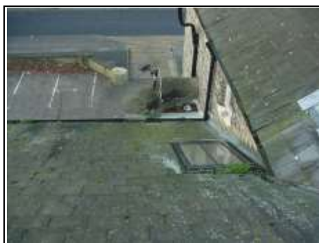
Roof light five – left hand side This is an awkward detail with vegetation growing at the top that needs to be removed as part of your annual maintenance programme
