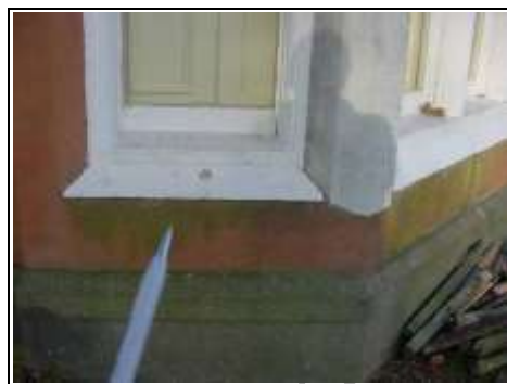
Movement in double bay to rear at low level
