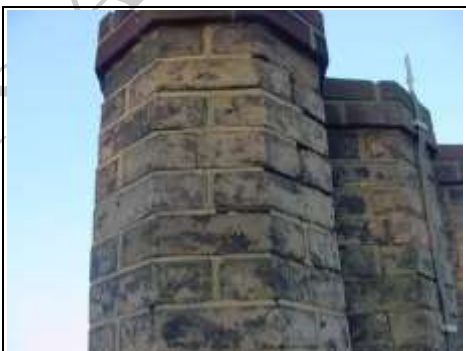
Close up showing cracking to brickwork and repointing required
