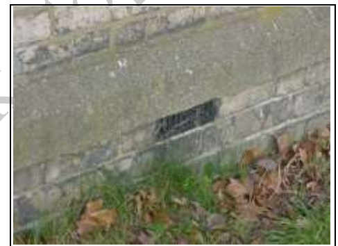
Airbricks that lead into cellar
