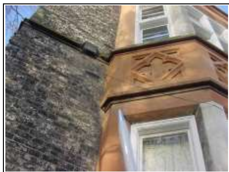
Movement in double bay to rear at high level
