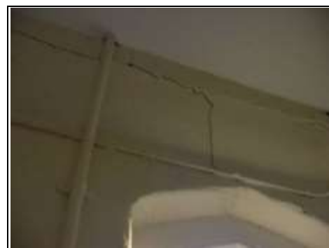
Cracking to lobby at top of spiral staircase
