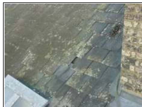
Missing slate to front left hand roof
