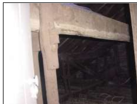
Woodworm to front left hand side roof
