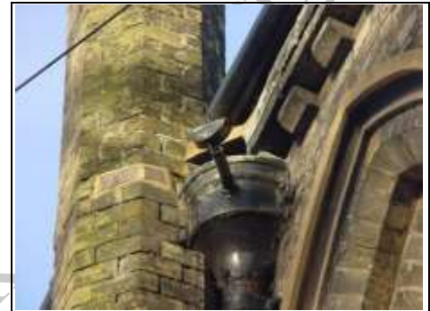
Hopper head overflowing, chimney needs repointing
