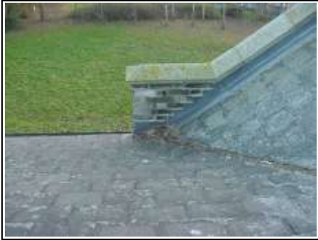
Blocked valley gutter
