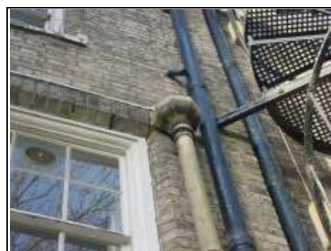
Lead pipework
