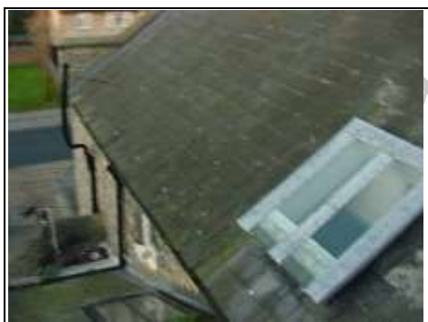
Roof light four – left hand side Older style wood made roof window which has then been covered with lead of equivalent and tends to be more problematic than the purpose made windows
