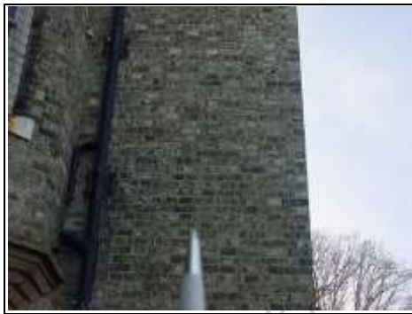
Vertical cracking to right hand wing
