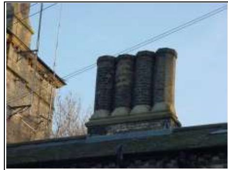
Minor spalling brickwork
