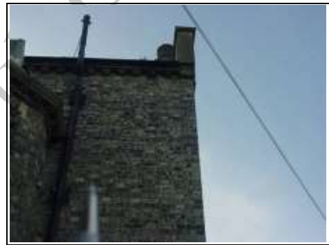
Vertical cracking to right hand wing
