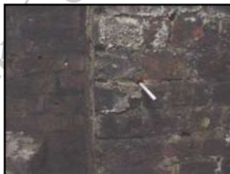
Pen indicates an example of one of many holes drilled in the wall in the basement
