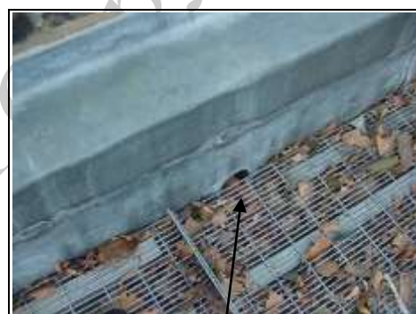
Example of how the box gutter gets blocked with the arrow showing where the outlet is in the parapet wall to the front of the property
