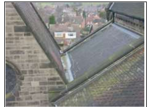
Valley gutter to north east roof
