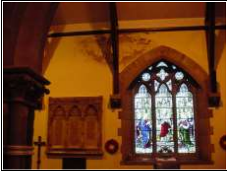
South aisle with efflorescence and dampness at high level
