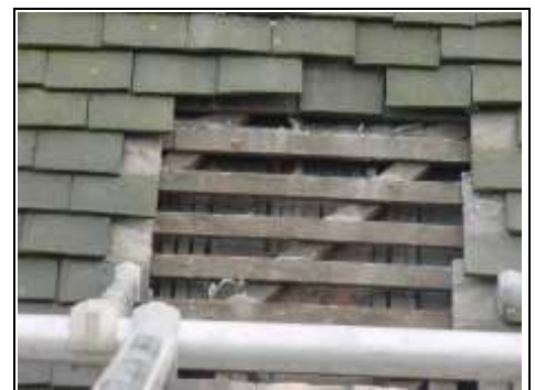
Battens and underlayer exposed on north elevation high level roof
