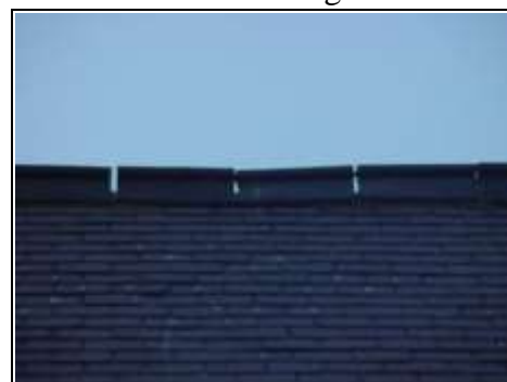
Overview of slipped slate to the south elevation
