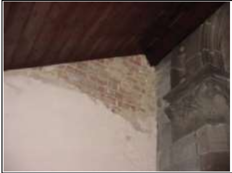
Dampness has caused the plaster come away
