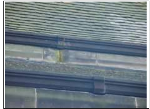
Leaking gutter sitting on a wall.
