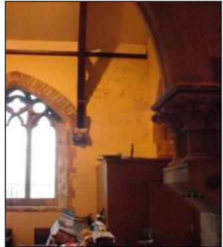
Front of the south aisle with efflorescence at roof level
