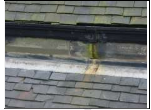
Leaking gutter
