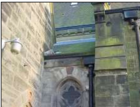
Overflowing valley gutter to north door entrance
