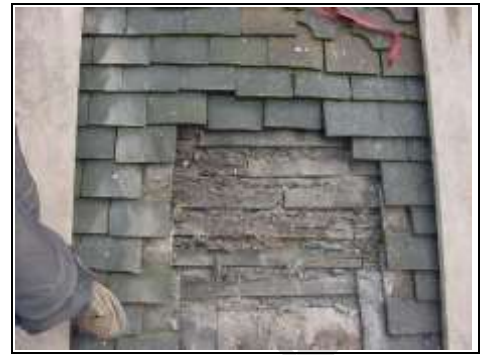
Exposed area on the Nave roof.
