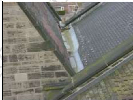
Valley gutter with lead tingles to the central area
