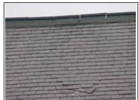
Slipped slates and deteriorating ridge tiles.
