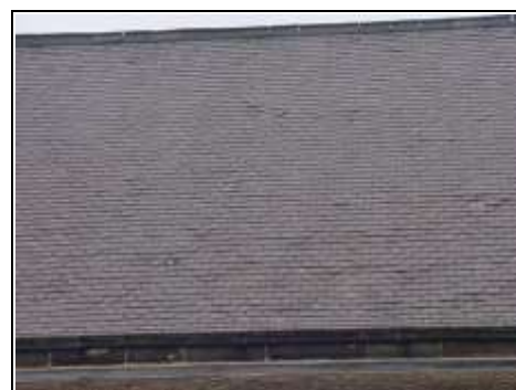
Close up of ridge, needs re-bedding
