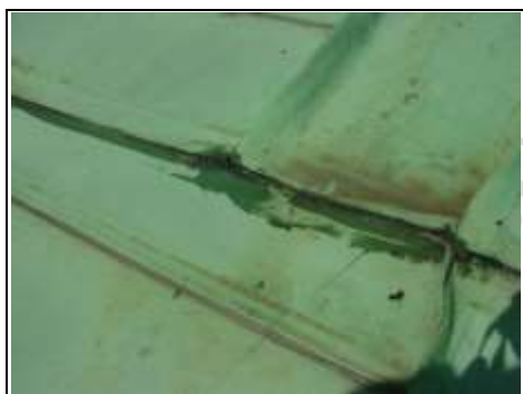
Poor quality mastic repairs
