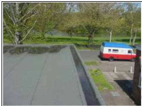
Rear flat roof showing internal gutters blocked and ponding
