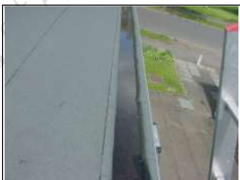
Rainwater sitting in internal gutter
