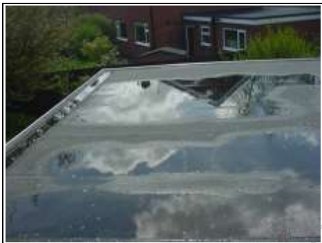
General view showing ponding
