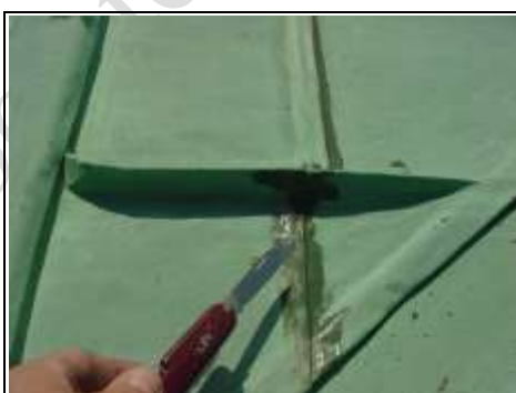
Example of painting over the joint rather than opening it up and carrying out a repair
