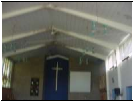
Concrete portal frame visible
