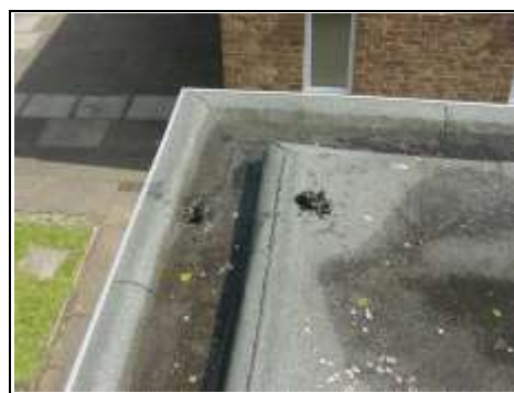
Rear flat roof gulley left hand corner which we unblocked during the course of our survey
