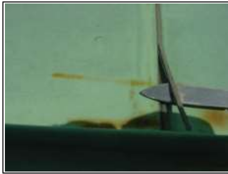
Original seals starting to deteriorate
