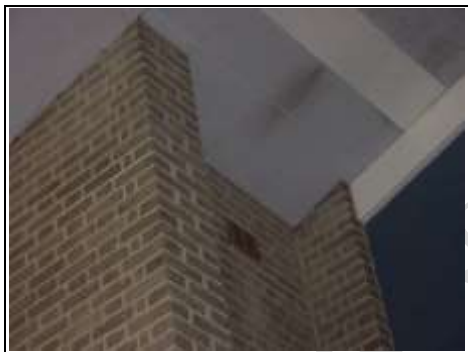
Front high level air vent
