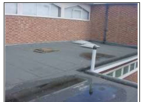
Excessive ponding and rainwater in internal gully
