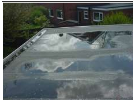
Excessive ponding front right hand side flat roof
