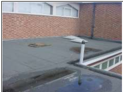
Rainwater sitting on the roof and in the gulley's
