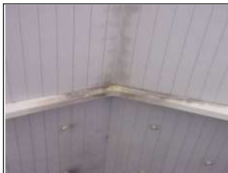
Black staining to portal frame, cold bridging
