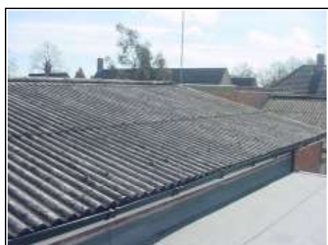
Asbestos roof. We believe that you have had an Asbestos Report carried out on the property as a whole
