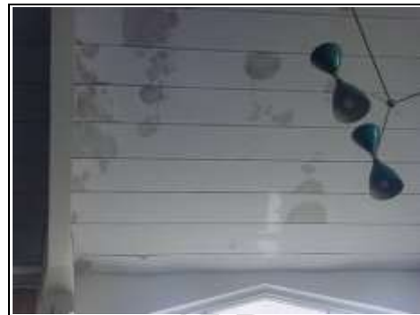
Spot/patch staining to the roof
