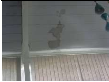
Staining to the roof
