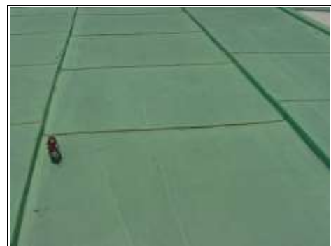
Horizontal lap joints
