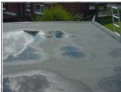
Ponding on flat roof
