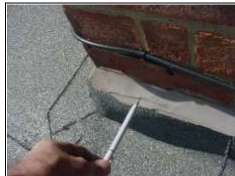
Felt flashing
