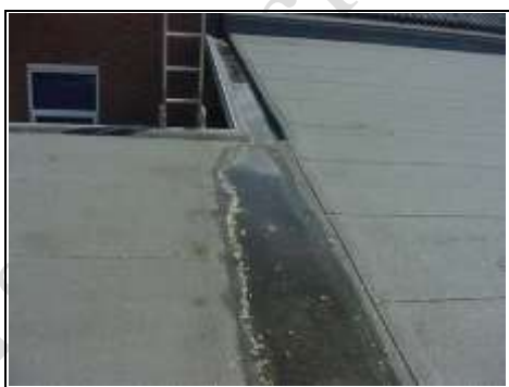
Rainwater sitting in internal gulley
