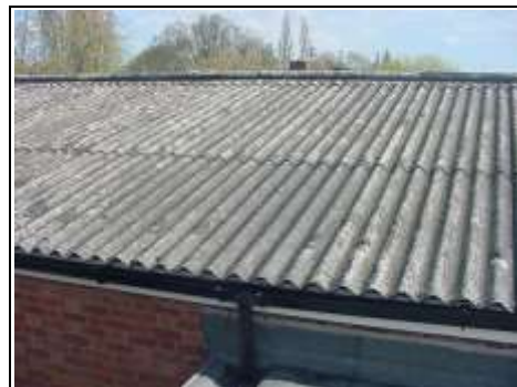
Newish profile shaped plastic gutter
