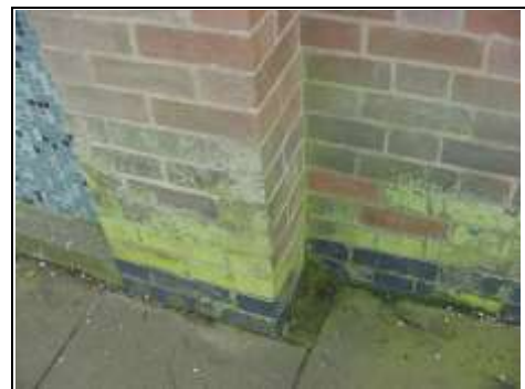
Greening of brickwork to the left hand side
