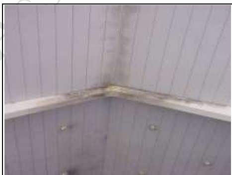
Cold bridging to portal frame and also to the ridge of the roof
