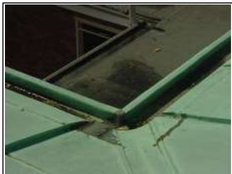
Mastic repairs to main roof internal gutter
