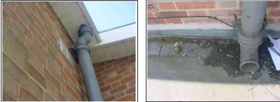
Cast iron downpipe
