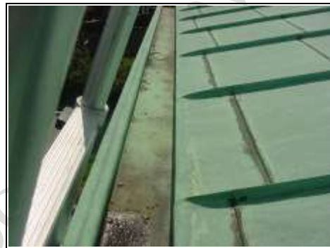
Internal gutters are relatively clean and show that there is a fall and no ponding within them (unlike your flat roofs)
