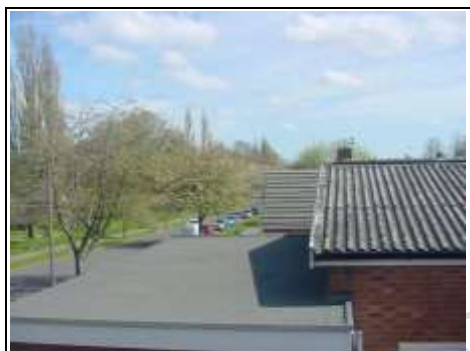
Partly flat roof partly corrugated asbestos roof
