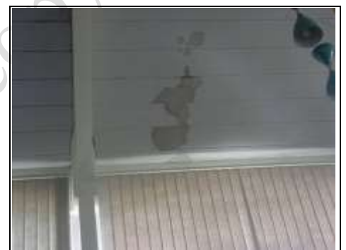
Patch/spot staining to ceiling
