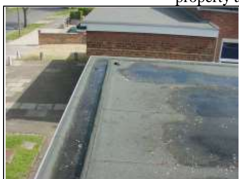
Blockage causing rainwater to sit in internal gutter
