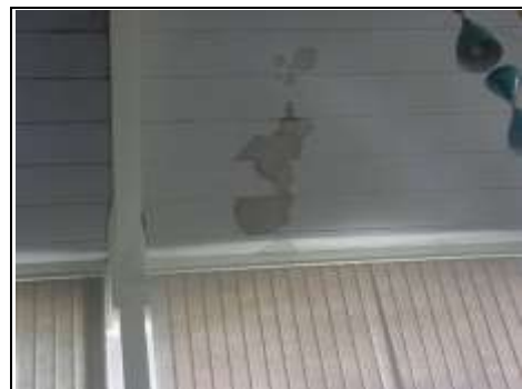
Patch/spot staining to ceiling
