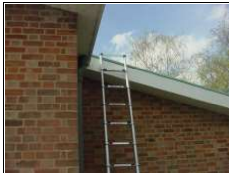
Overclad soffit
