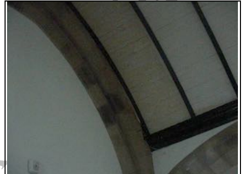
Difference in colour on barrel roof believed to be due to dampness in this area
