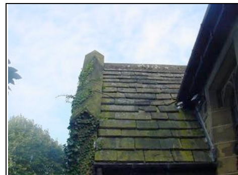
Damaged stone slabs to roof
