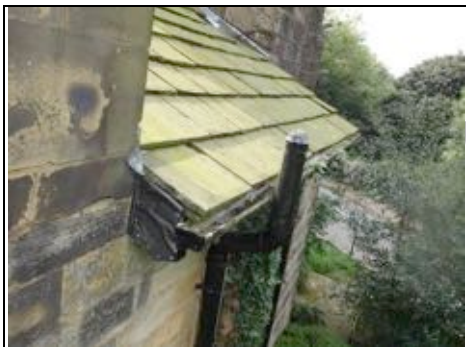
DIY plastic repair to fascia board
