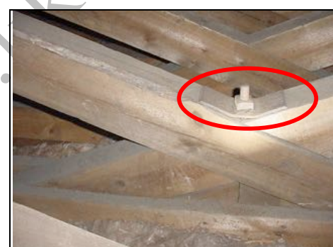
Bolt at top of horizontal tie bar
