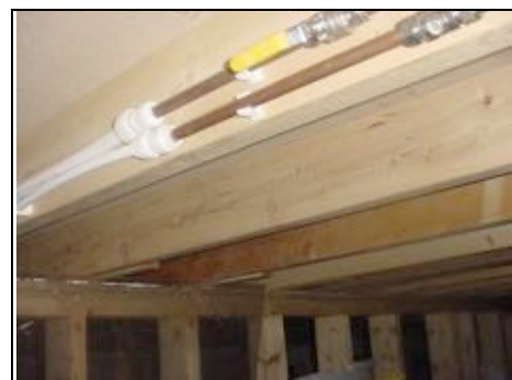
Mix of plastic and copper pipes under the lounge
