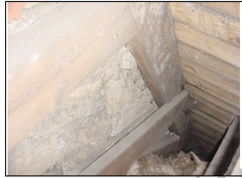
Wall between the Nave and Chancel with brick to the top and stone down the side
