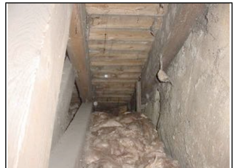
Close boarding and insulation
