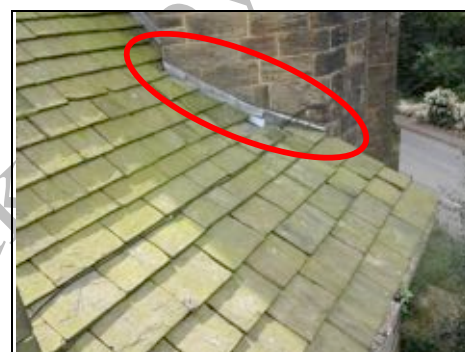
Flashing coming away around Tower
