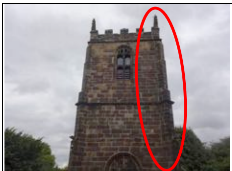
Lightning rod runs down to the ground
