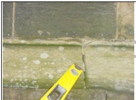
Weathering to stonework and deteriorating pointing
