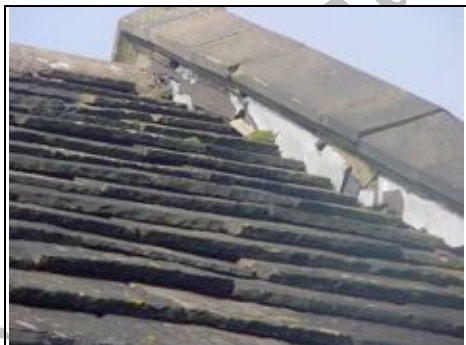
Flashband flashing deteriorating on chancel roof
