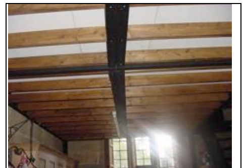
Underside of first floor, see how the steel beam twists with the timbers in it
