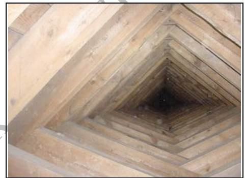
Timbers are in relatively good condition
