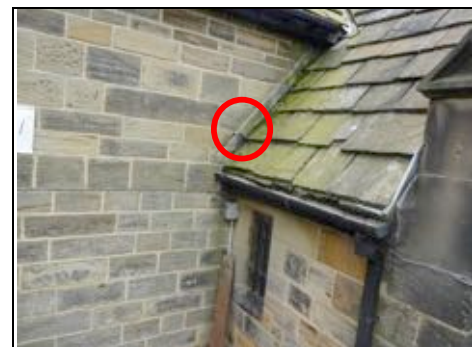
Extra lead added (red oval) and missing lead (green oval). Leadwork needed Aerial view – 360 photo
