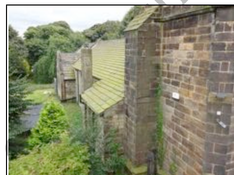
Roof adjacent to tower covered with moss
