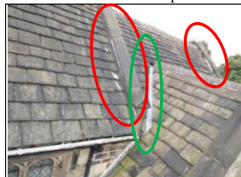
Two main parapet walls with Flashband repairs (red ovals) and valley gutter (green oval)
