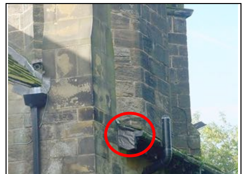
More Flashband repairs
