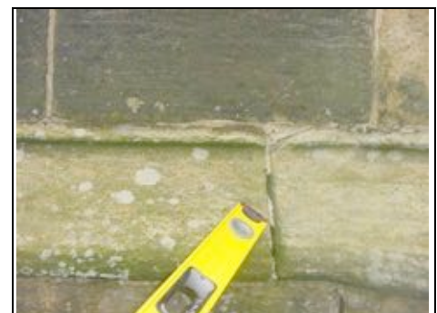
Weathering to pointing
