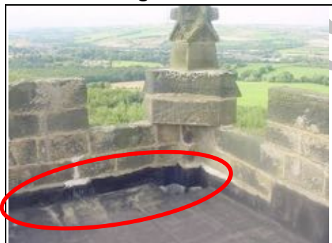
Problems with flashing on roof
