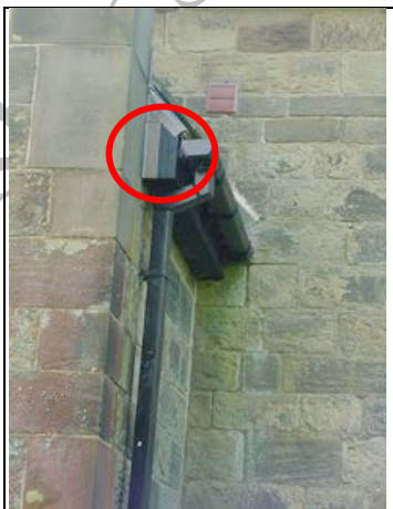
Flashband repair to fascia on north side
