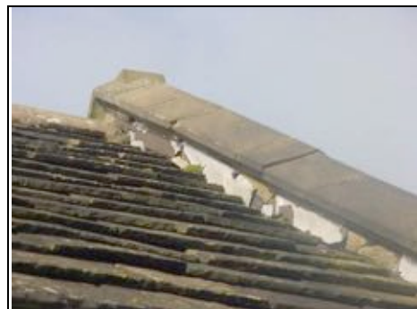
Deteriorating flashing on parapet
