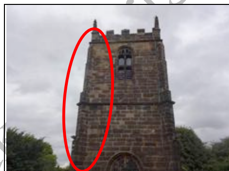
Water discharges down Tower
