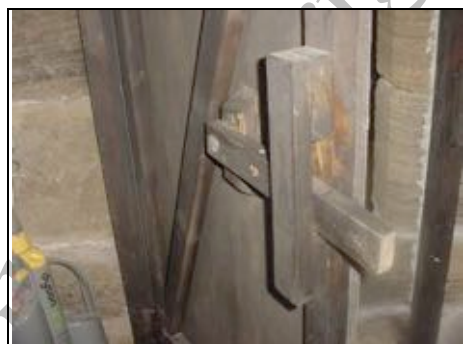
Lovely old fixings, including this latch to the door in the Tower doors
