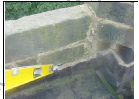
Pointing coming away from the flashing
