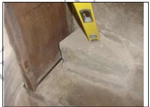
Stone steps to west side of Tower, level indicating new bit of stone added, meaning the door can no longer open
