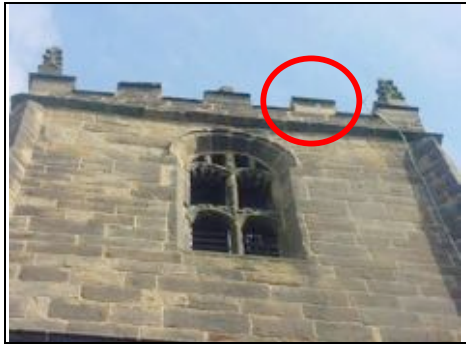
Old repairs to parapet visible
