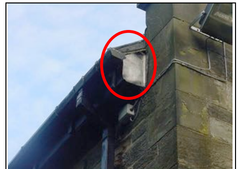
Flashband repair front right side
