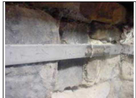
Close up view of the bracing bar
