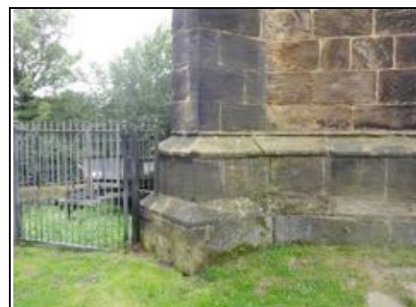
Water runs to the base where there is worn out pointing and deterioration to stonework
