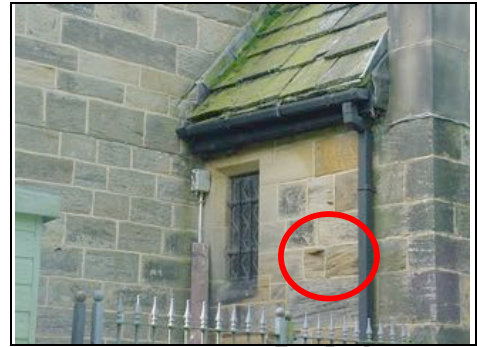
Damaged stonework to north side
