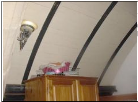
Barrel ceiling / waggon roof
