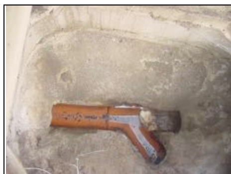
Manhole slightly blocked
