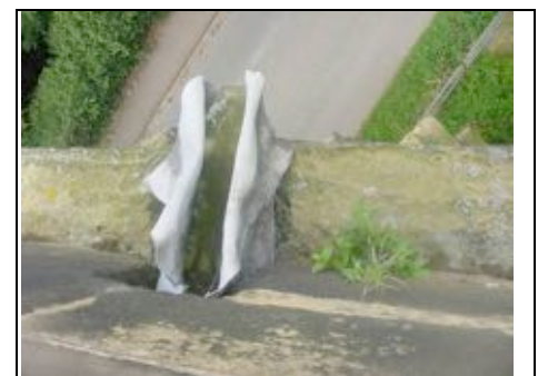
Rainwater gully discharges rainwater down wall
