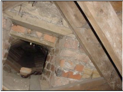
Over Chancel Arch where there is a mixture of brick and stone
