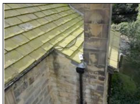
Base of chimney, with overflowing hopperhead to the side.
