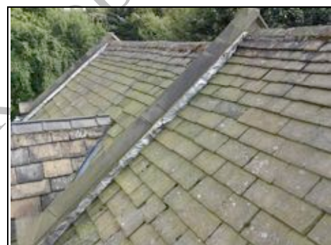
Flashband repairs on parapet
