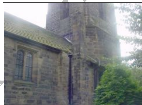
Hopper head and gutters discharge
