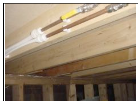
Mixture of plastic and copper piping
