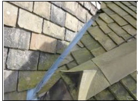
Repairs to valley gutters Aerial view – 360 photo
