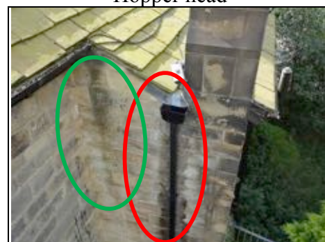
Leaking hopper head– staining down wall (red oval) and overflowing gutter (green oval)
