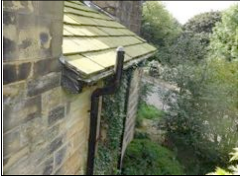
Soil and vent pipe to rear left
